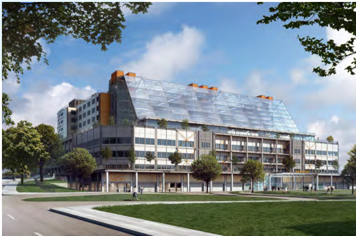
Midland Metropolitan Hospital Image source: www.swbh.nhs.uk
